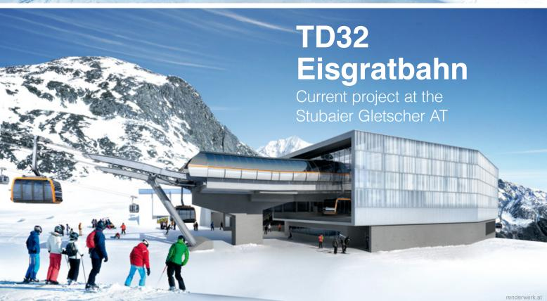
The tricable gondola lift "3S Eisgratbahn" will be in operation throughout the year. It will meet the highest requirements in terms of performance, cost-effectiveness and environmental sustainability and represent a new generation of technology. The installation will be the first tricable gondola lift realized in two sections and to use the environmentally friendly DirectDrive.
