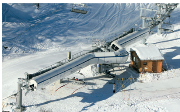
Single-sided middle station with boarding and deboarding (CD6 Nationale Express)
