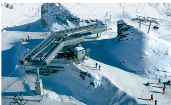
Middle station as “top station” (TMX6/8 La Chaux Express)
