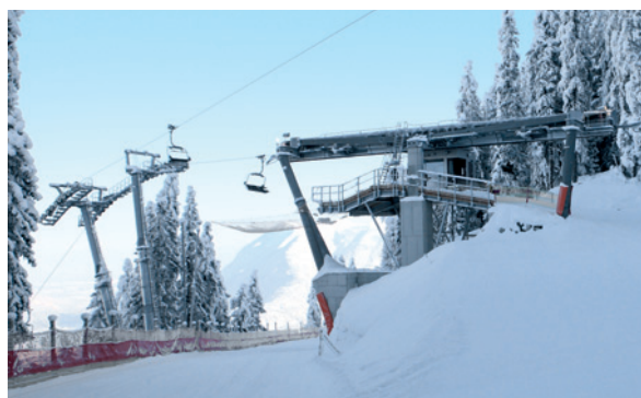
Single-sided deboarding station (CD4 Kandahar Express)
