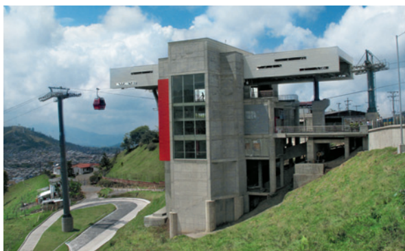
Middle station of a “multiple-section ropeway” with boarding/deboarding (GD10 Cable Aéreo Manizales)
