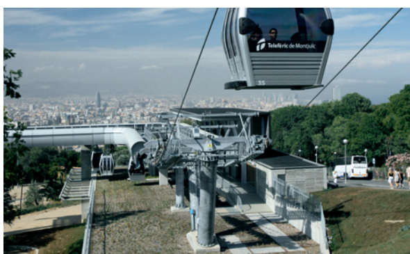
Middle station with 90° deflection (GD8 Teleférico de Montjuïc)
